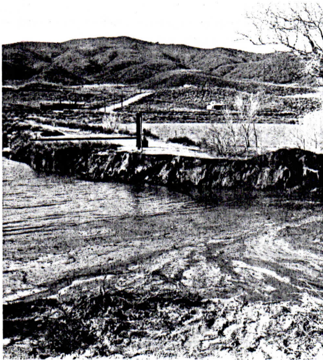
North end of dam after cut. Soon to be restored.
